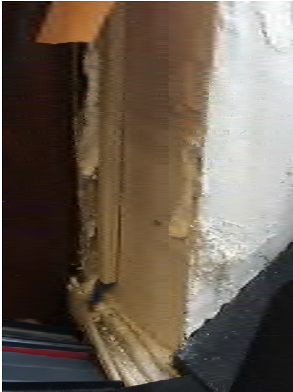
DETERIORATED PLASTER AT WINDOW JAMB
