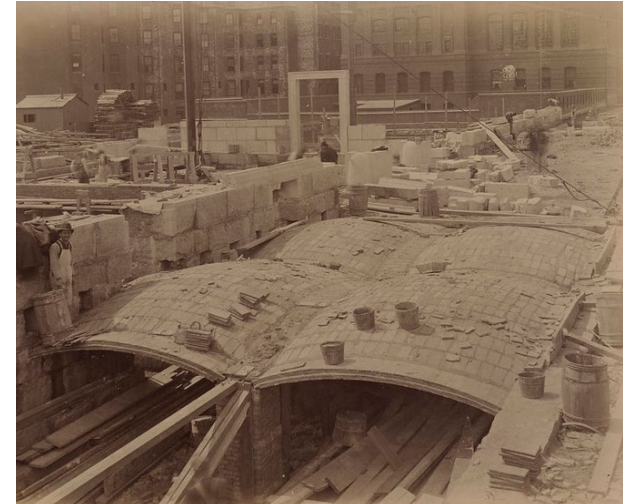
Basement Construction of Guastavino Arches
