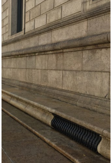
Edge seating with integrated exhaust vents
