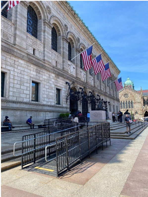
Existing Temporary Ramp
